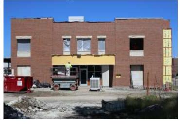
Construction continues to move steadily on the new Sedalia Police Headquarters. All stair pans have been filled with concrete and much of the building's gypsum and tile backer board is in place. Most notable for the passer-by is the brickwork and installation of the west canopy on the outside of the building. Window measurements have been taken in anticipation of installing the glass once brickwork has been completed. Building completion date is still estimated for mid-November.
